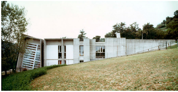
Figure 3. Eastern facade. Sergio Los and Natasha F. Pulitzer, Kindergarten, Crosara, Italy, 1972–78. (Source: Synergia Progetti archive: Sergio Los, Natasha F. Pulitzer).
